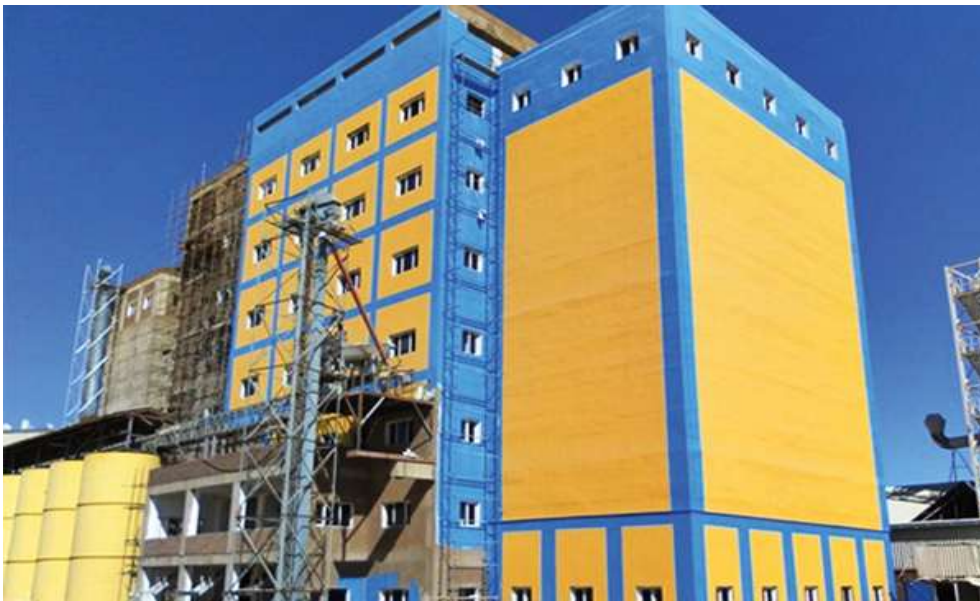
Figure 1: A 2 Mill Installations from Ugur Group in Sudan
